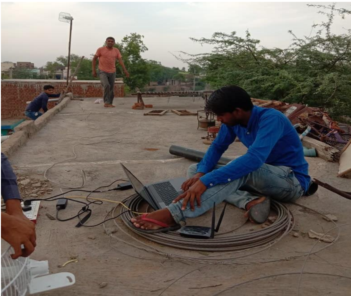
Installation of Community Network by Wireless Trainers in Nuh, Haryana
