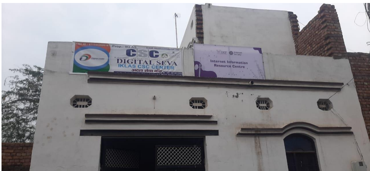
Tower installed at Tauru Internet Information Resource centre, Haryana
