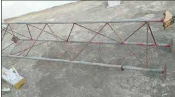
Figure 4 Example of showing 10 feet long tower using three pipes
