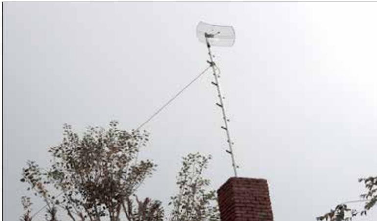
Figure 10: PVC pipe with GI wires
